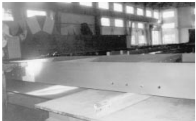
Fig. 4 Arc-sprayed Al coatings were applied on the bolting surface of Wuhu Yangtse River bridge
